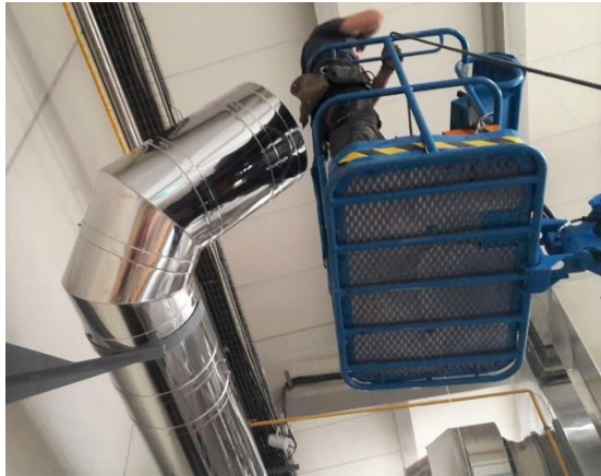
No heavy lifting
