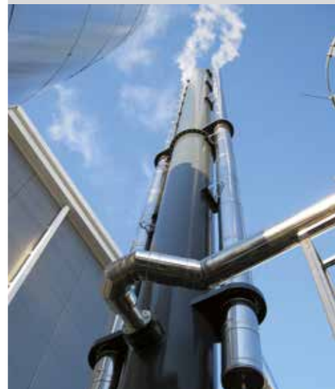
Flange connection secured by internal V-band and locking band 2.0 in the external.
