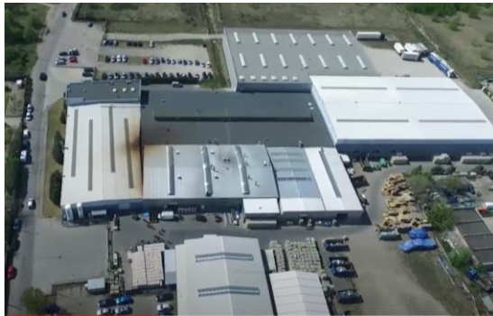
Production site Poland
