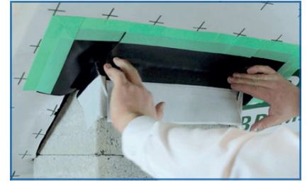
Inner corner can be plastered over
