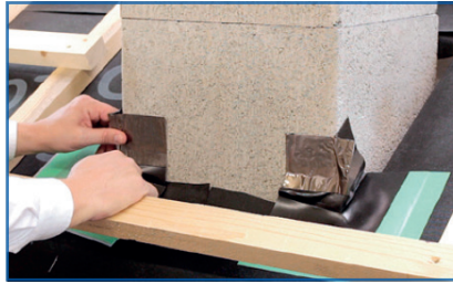
Inner corners plastering not possible
